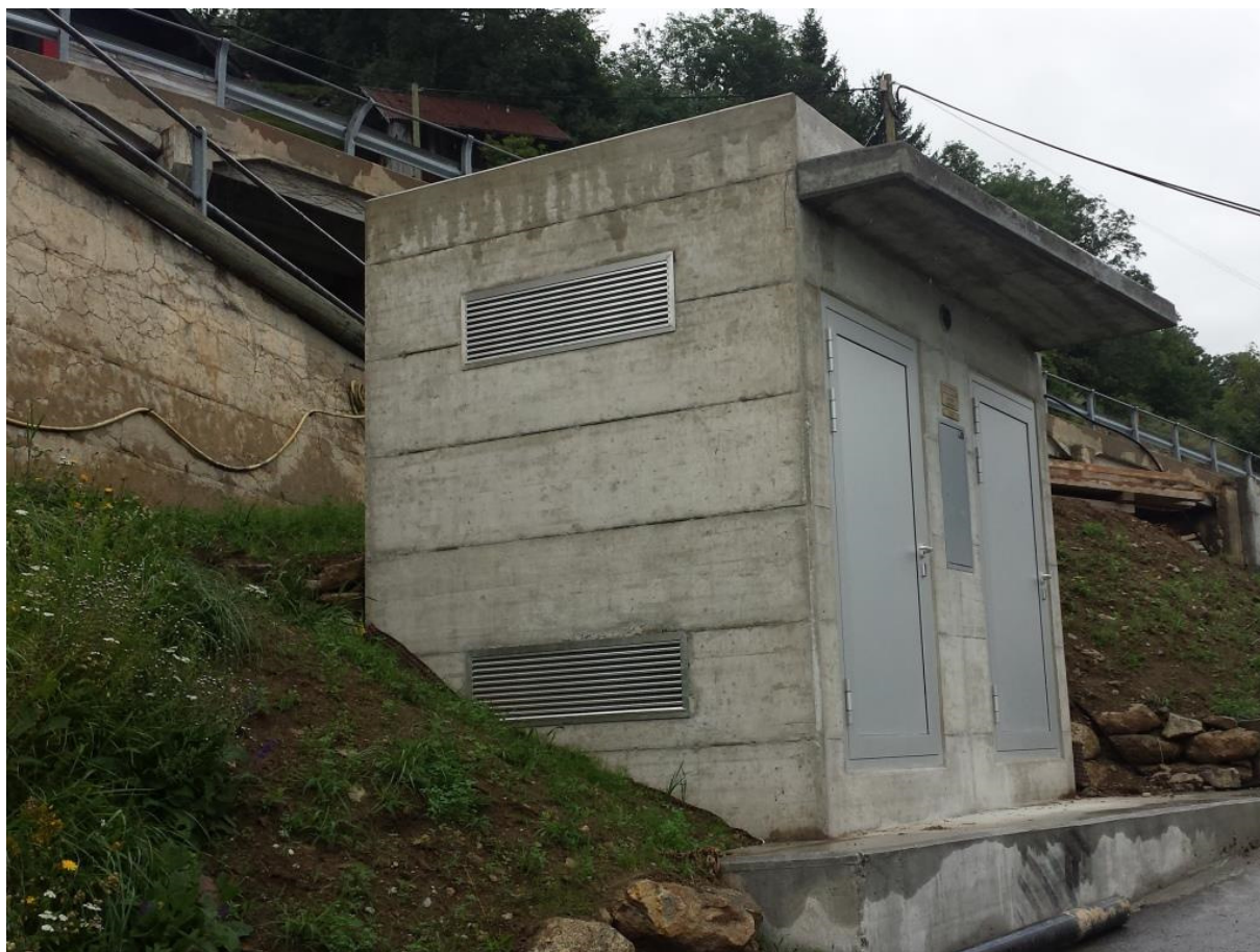
Neue Trafostation Eggen in Eggerberg
